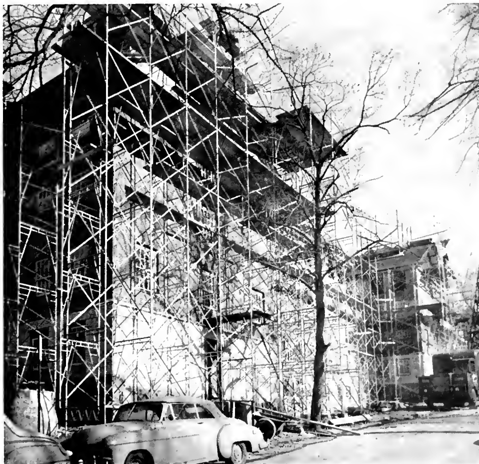
BUILDING'S height is suggested in this view up Charles Field St.
